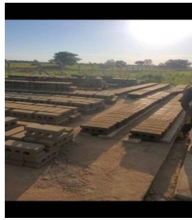
Bricks being made by missionary Baxter for construction
